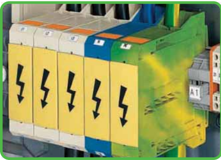
Protective warning marker may indicate: Caution! Power is still on even after switching off the main switch!
