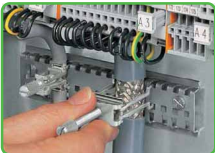
Fitting an additional clamping saddle.
