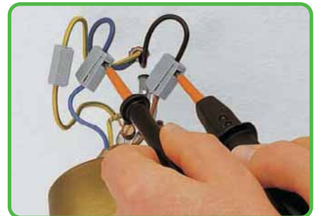
Testing through separate test slot.
