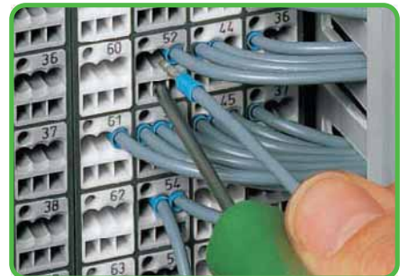
Terminating ferruled conductors.
