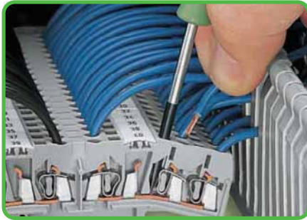
Terminal blocks for matrix patching. Conductor termination/removal on the terminal block's side-entry.
