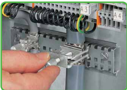
Tightening/Removing a clamping saddle.
