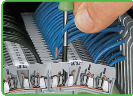
Terminal blocks for matrix patching. Conductor termination/removal in center of the terminal block.
