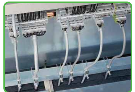
Cable entry in the base of the switch cabinet, with separate strain relief, movable IP54 bottom plates sealed with sponge rubber (e.g., by Rittal)
