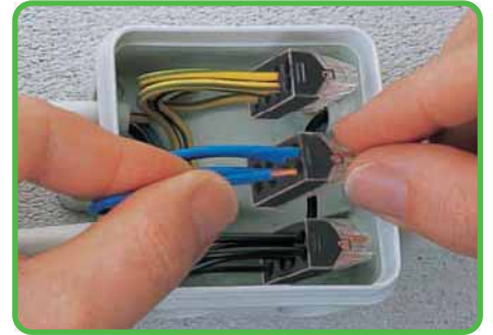
Termination: Insert stripped, solid conductor fully.
