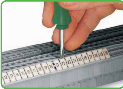
Snapping a strip into the marker slot.
