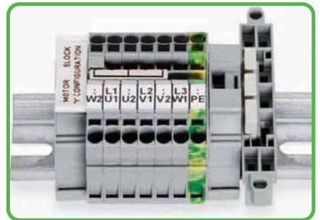
Star point jumpers designed for 'Y' configuration
